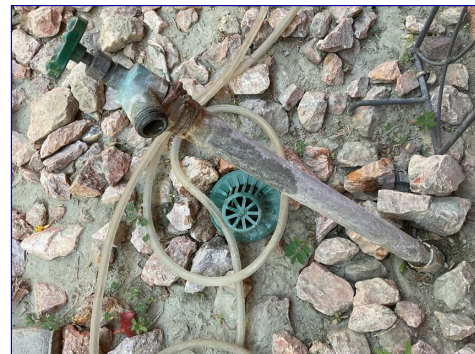
Recommend reinforce the hose bib piping.
