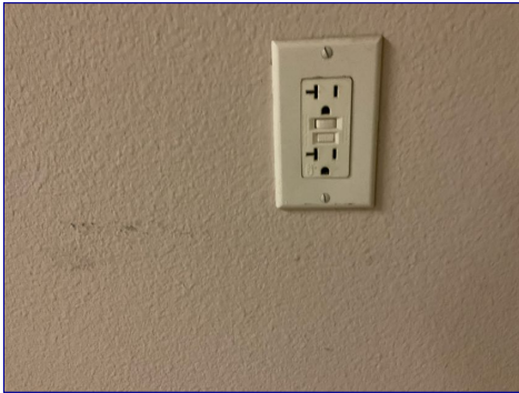
No reverse polarity or open ground.
