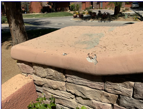
Some of the trim was damaged. Recommend repair or replacement of damaged exterior trim by a licensed contractor.
