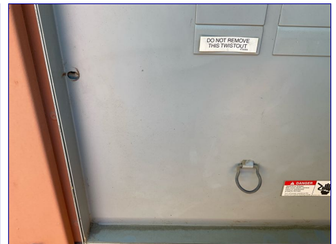
Missing screw on left side of panel. Recommend replace.
