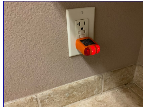
GFI installed. No reverse polarity or open ground.
