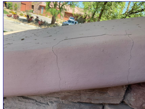
Some of the trim was damaged. Recommend repair or replacement of damaged exterior trim by a licensed contractor. Location front right side by gate.
